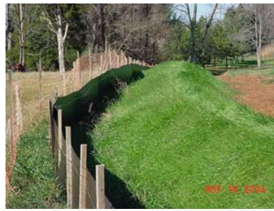
Stabilization of construction sites prevents siltation of waterways
